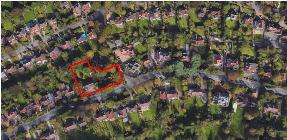
Figure 2: Aerial View for the site's location.
